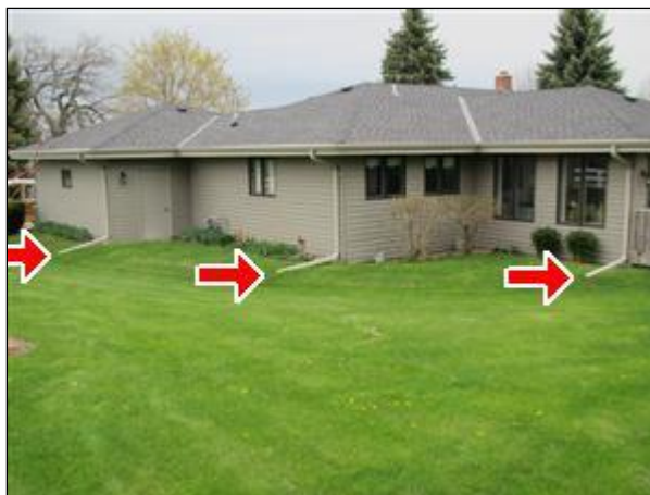
3.0 Picture 1 Drainage Swale
