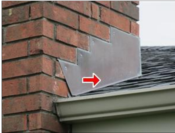
1.1 Picture 1 Copper Flashings
