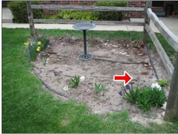
5.1 Picture 1 Holding Tank Cover Buried Here
